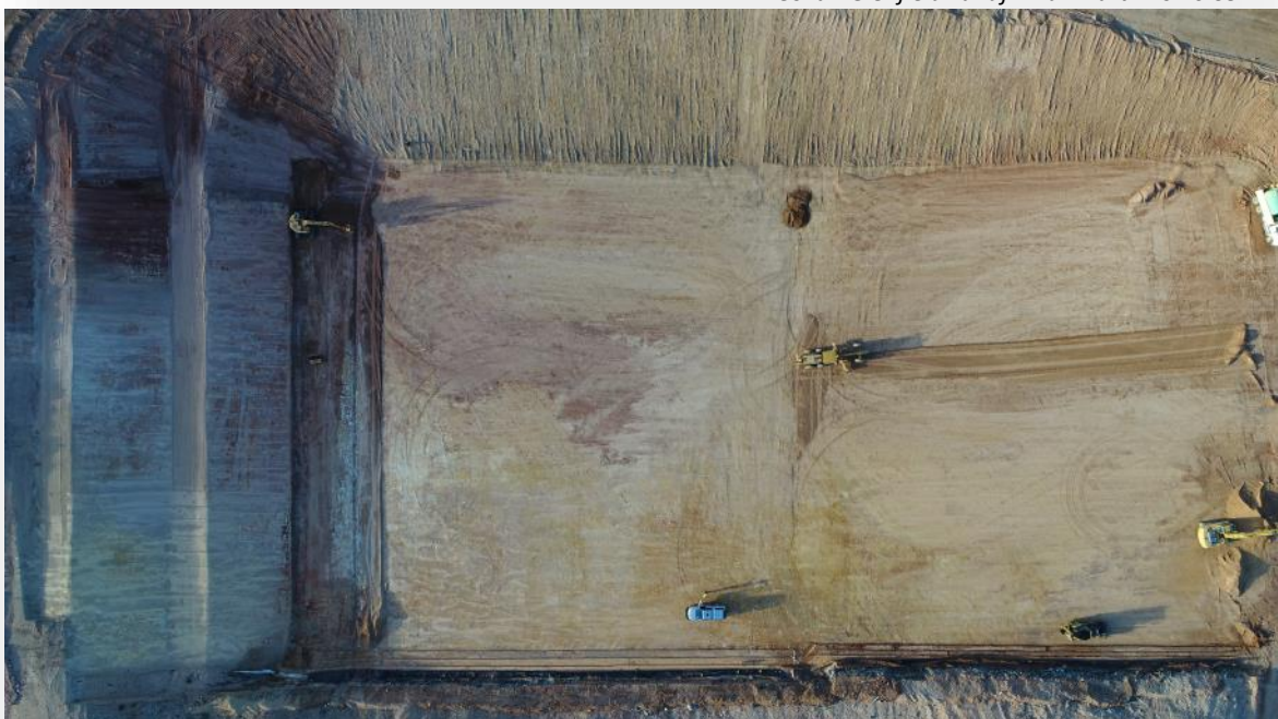
Veolia - Glenfield Landfill Bulk Earthworks Cell 2
